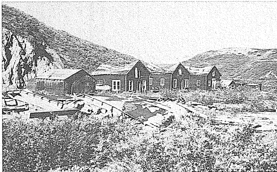
Abandoned structures at the Dunkle Coal Mine in Denali National Park, 1981.
