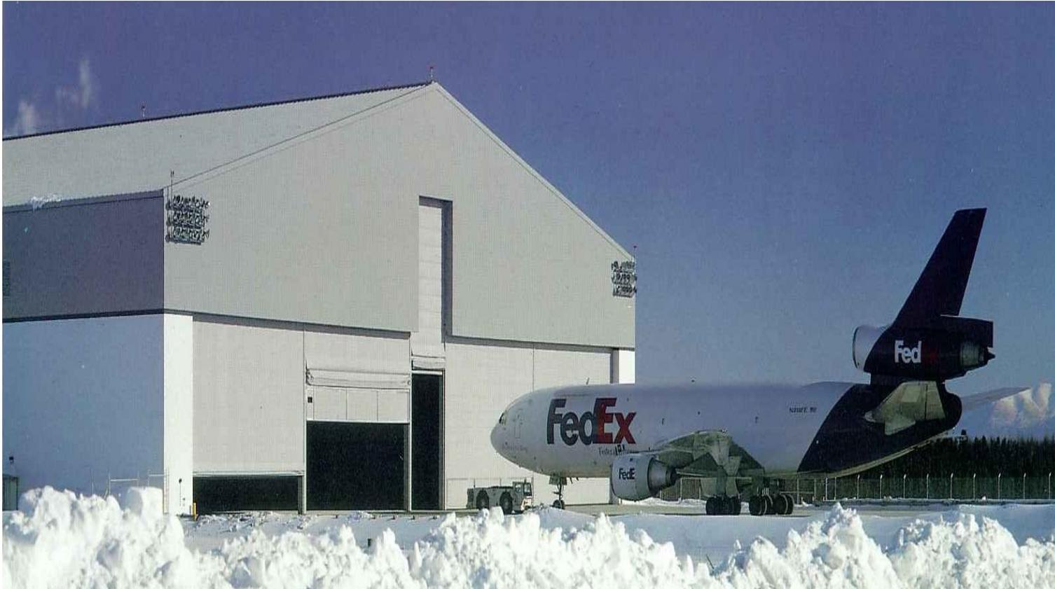
The Federal Express Maintenance, Repair and Operations (MRO) facility consists of a hangar capable of accommodating one wide-body aircraft, such as a Boeing 747. The project also includes a ramp, taxiway, road, utilities and landscaping. The hangar is supported by a fire suppression pump house and water storage facility, which was
