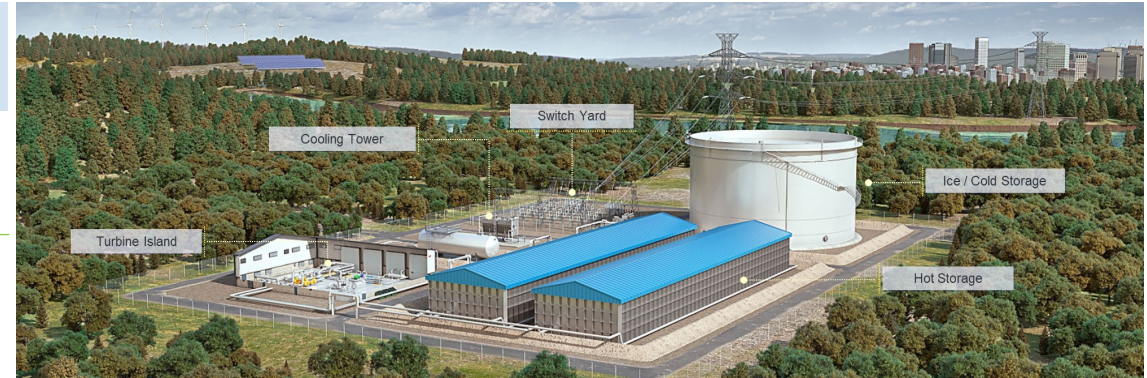
Nominal system size 1,000 MWh: 100MW, 10hr on less than 6 acres
