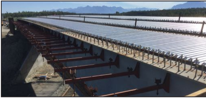
Parks Highway MP 47.5 Bridge – Orion Marine Contractors, Inc.
