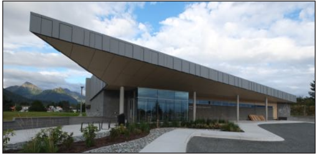
Mt. Edgdecumbe High School Aquatic Center – Cornerstone General Contractors, Inc.
