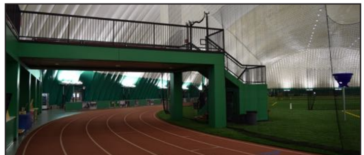
The Dome/Reconstruction – Davis Constructors & Engineers, Inc.
