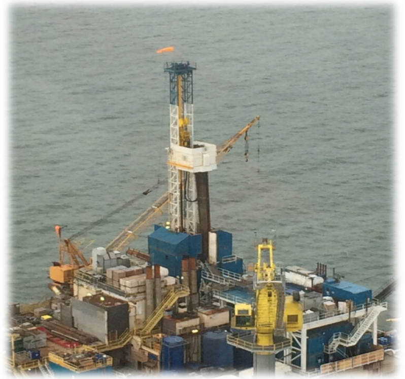
King Salmon Platform – Kuukpik 5 Rig
