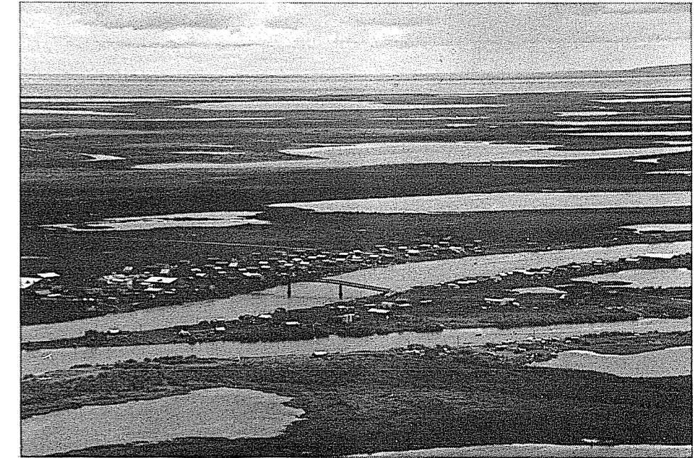
The village of Selawick, like many in Alaska, is built on wetlands near a navigable stream. A policy of "no net loss" for Alaska would create serious economic consequences throughout urban and rural Alaska and pose serious impediments to development projects in all resource sectors. (John Rense NANA)
