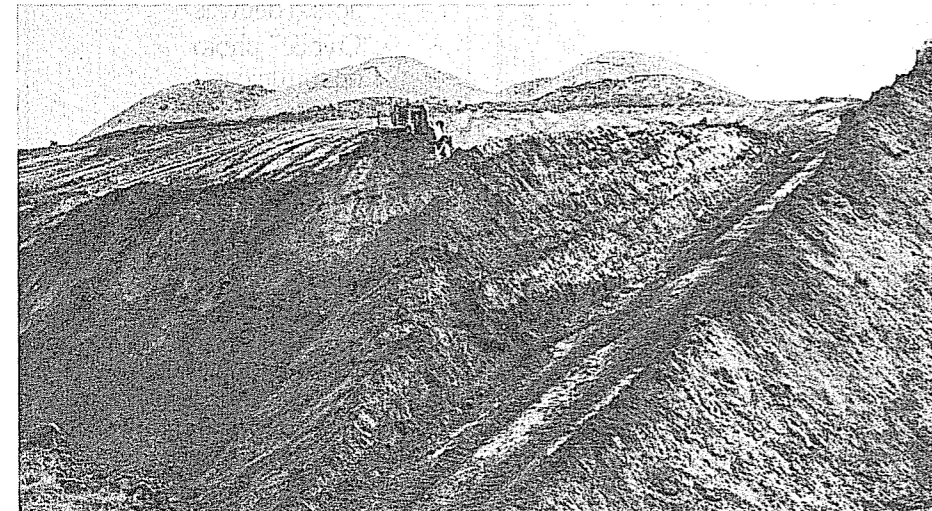
The initial reclamation stage involves regrading the disturbed land.
