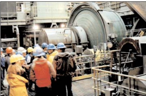
The Greens Creek ball and SAG mill receives ore from the mine. Here it is crushed and processed.
