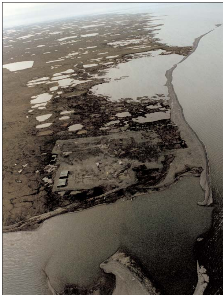
Point Thomson's central production facility pad would be located on the coast with two additional pads to the east and west. A 12-inch elevated pipeline would carry the gas condensate to existing infrastructure at Badami, 22 miles west.
