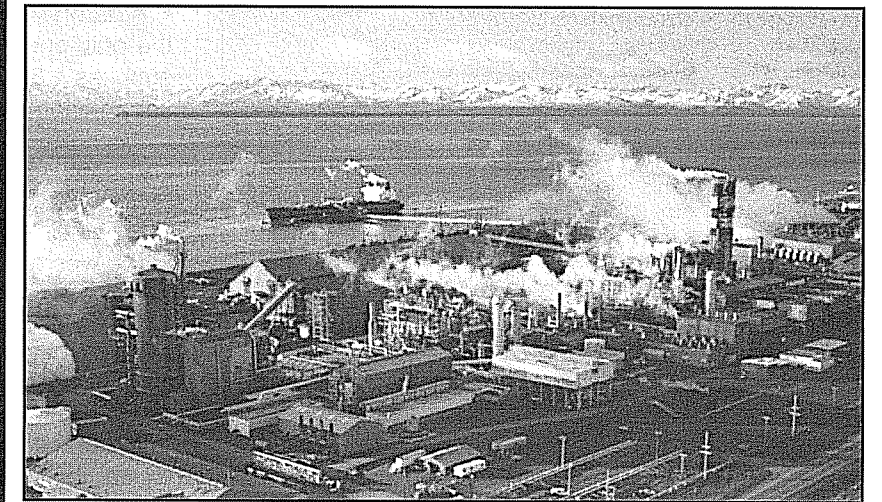
The Unocal chemical plant on the Kenai Peninsula uses Cook Inlet natural gas to manufacture nitrogen-based fertilizers.
