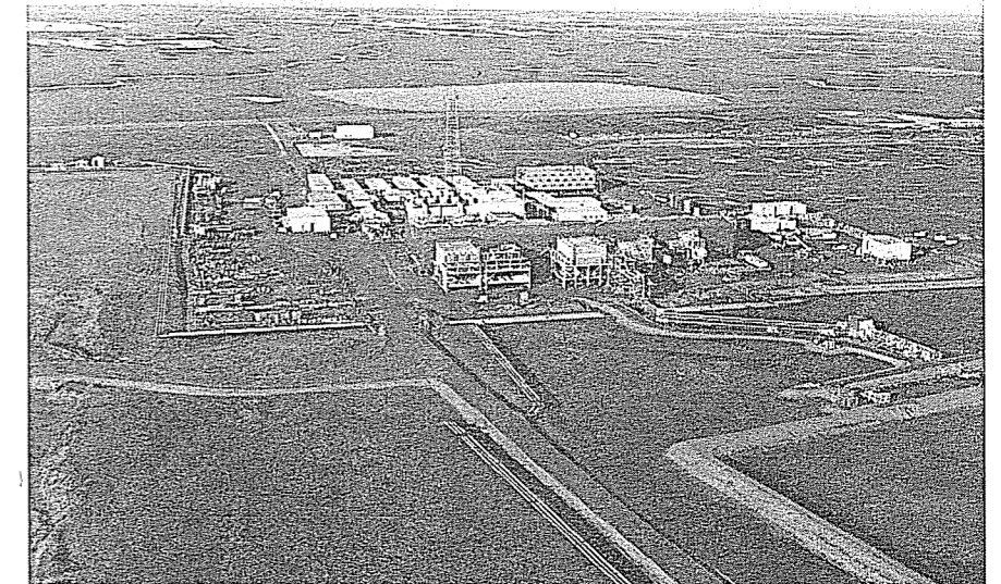
Although Alaska may hold over half of all oil and gas reserves to be discovered in America, industry activities within the state could be severely curtailed by increased regulations and cumbersome government policies.
