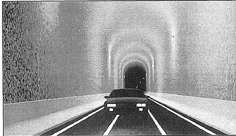
A computer simulation depicts an upgraded one-lane Alaska Railroad tunnel to Whittier. Both private vehicles and Alaska Railroad trains would share the 2.5-mile tunnel.
