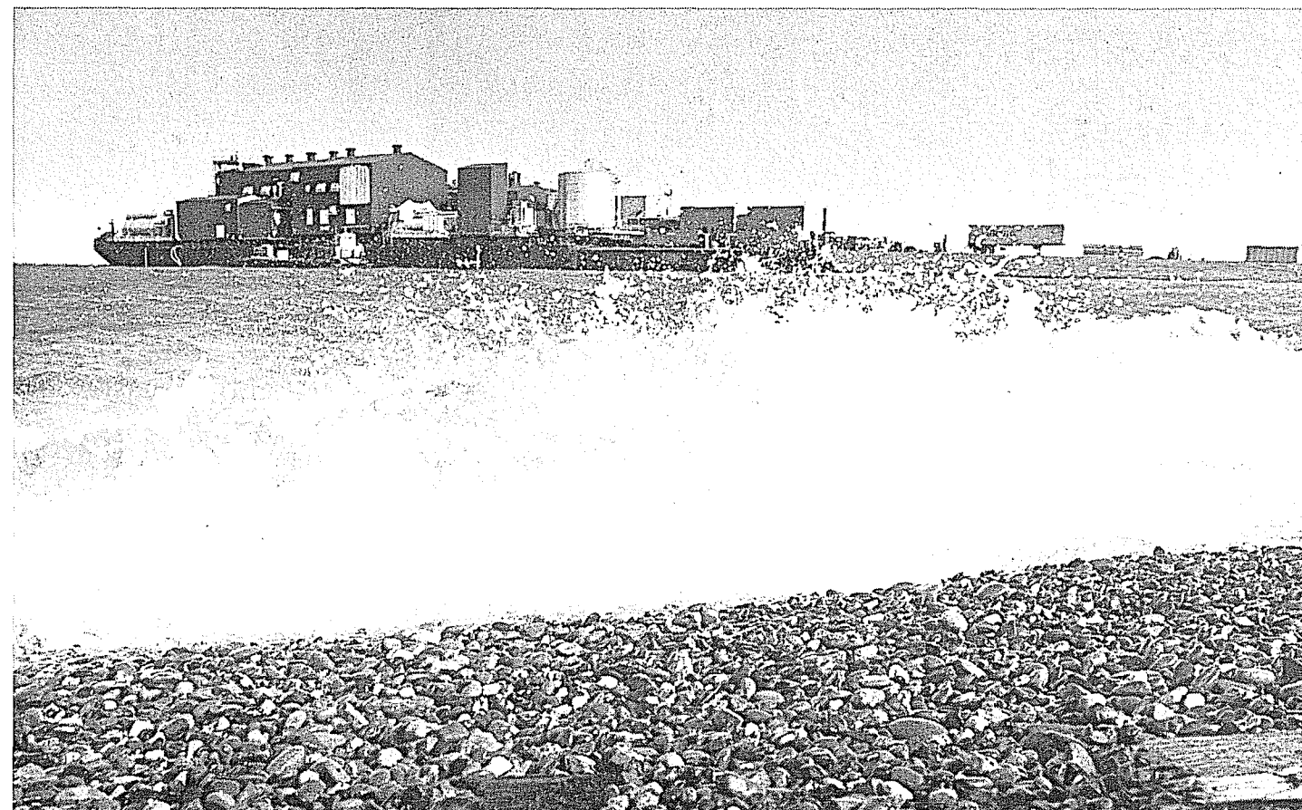
The construction of North Slope production facilities, including these giant modules, funneled millions of dollars into the national economy. These modules were transported by barge to the North Slope.
