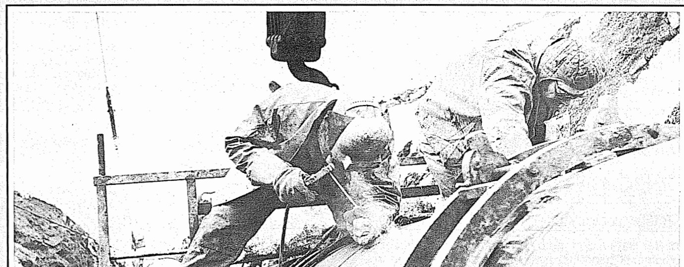
Pipeline welders complete the final weld for the Thompson Pass section of the trans-Alaska pipeline project.
