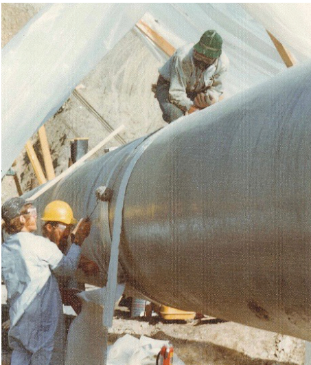
Crew insulates a joint on the pipeline north of the Yukon River in the summer of 1976.
