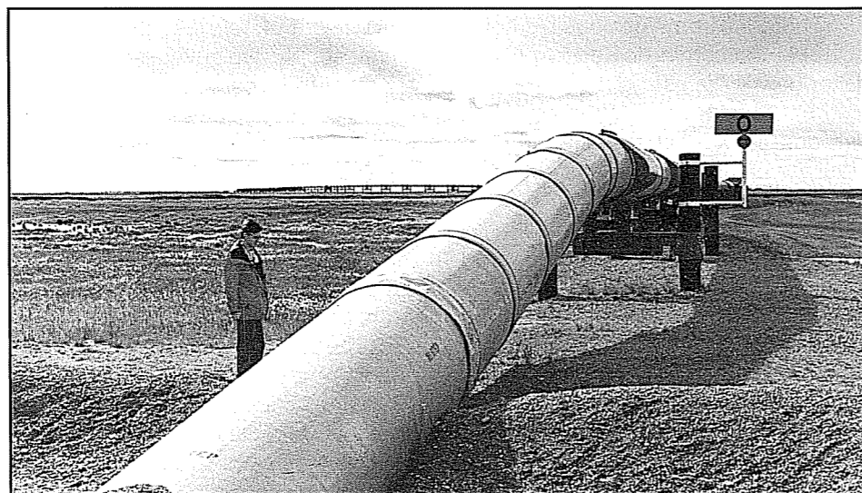
Milepost "O" at Pump Station 1 is where Prudhoe Bay oil begins its 800-mile journey to Valdez. More than 14,000 tankers have sailed from Valdez carrying 11.5 billion barrels of oil to U.S. markets. North Slope oil fields now account for 20 percent of domestic production.
